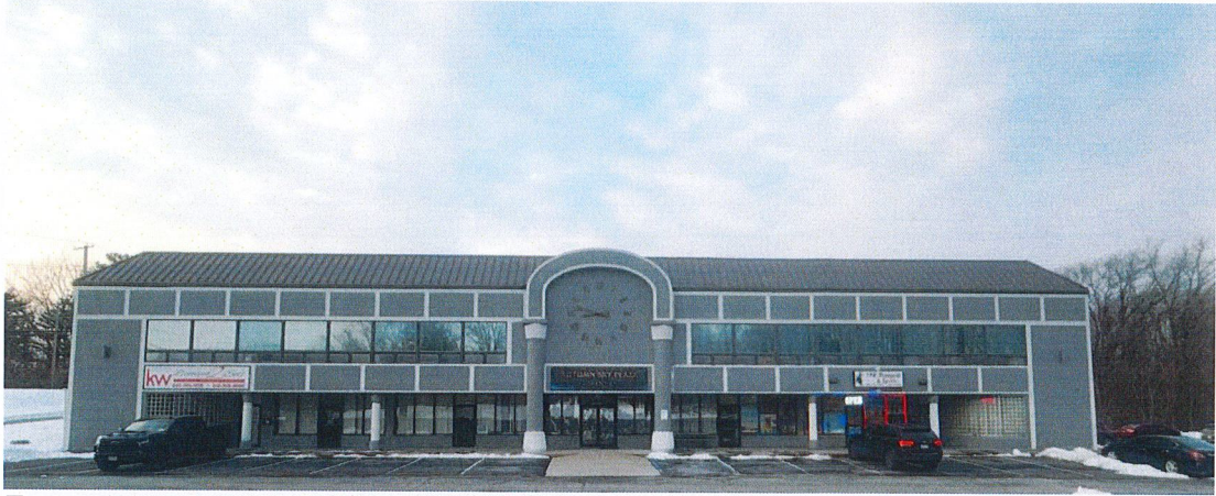
Existing Main Lower Level (Project Entrance)
