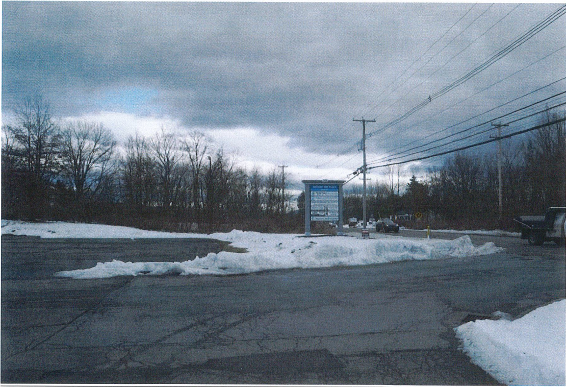
Existing Freestanding Street Sign at Entrance
