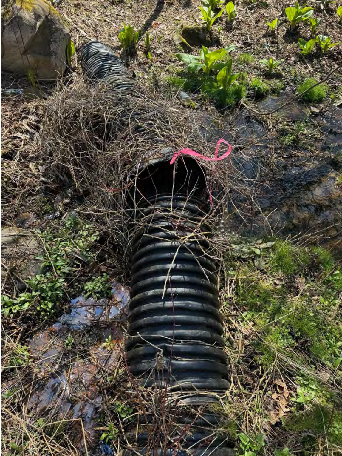
Attachment 1: Pipe Separating
