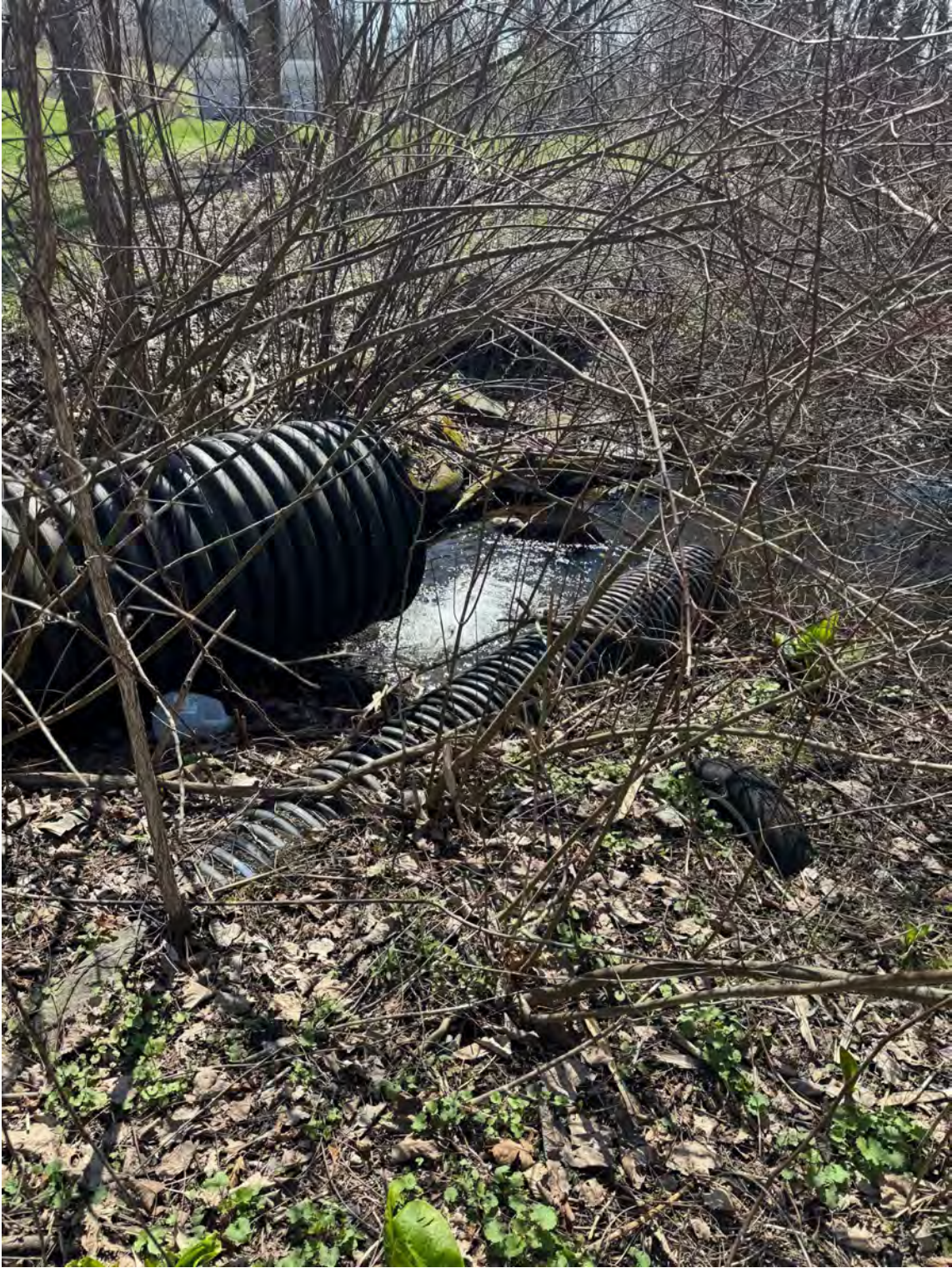
Attachment 2: Pipe Discharge 36" and 15"
