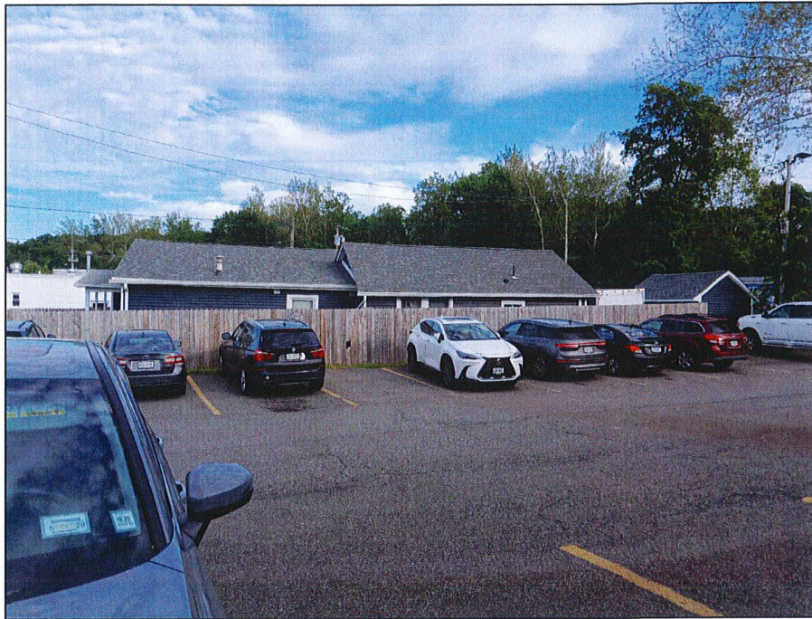
PICTURE # 5 EAST ELEVATION/RIGHT SIDE FROM TARSIO'S
