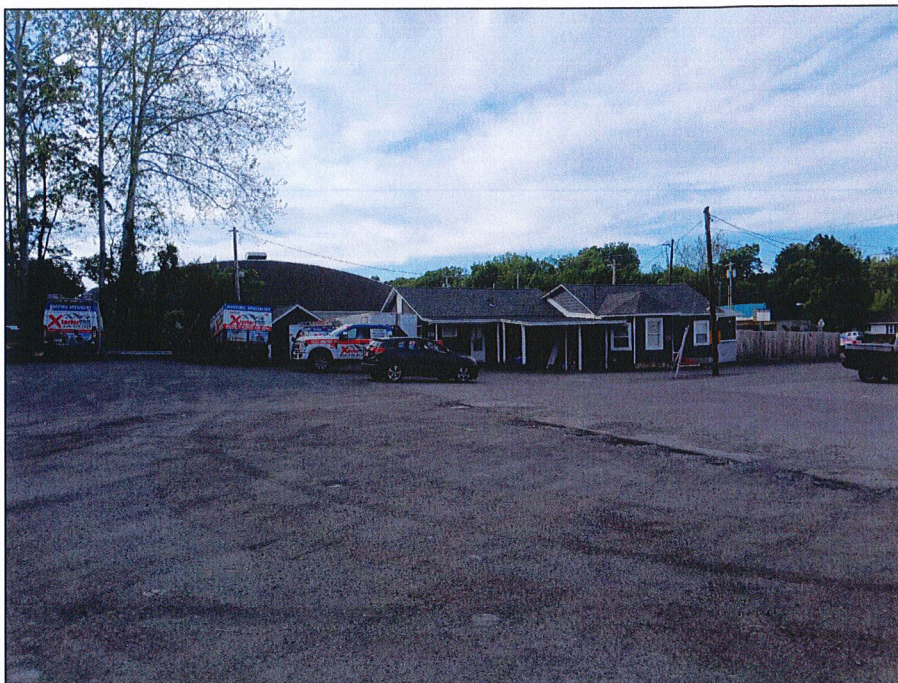
PICTURE # 7 WEST ELEVATION/LEFT SIDE FROM DRIVEWAY EASEMENT
