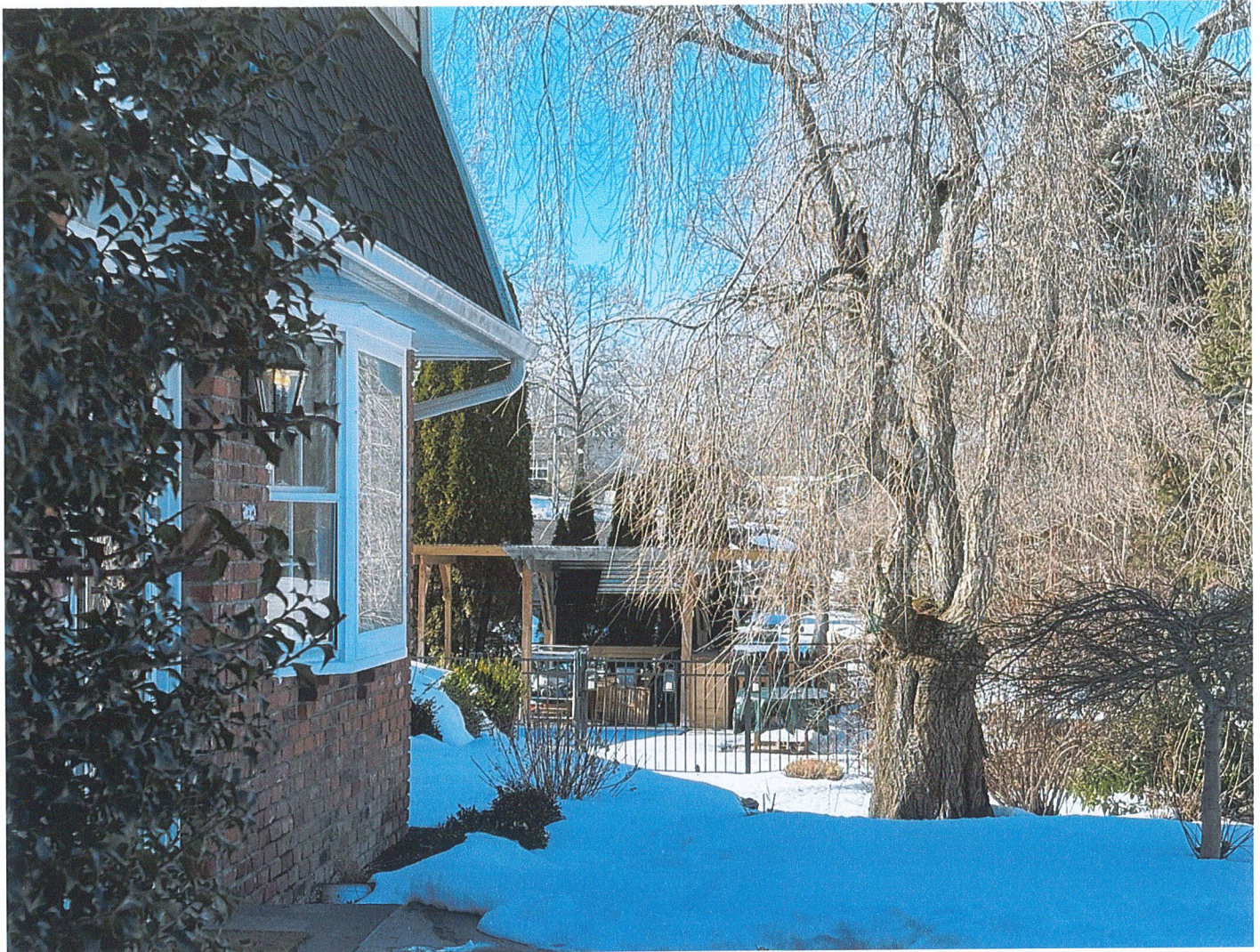
Photo 3: Fenced pool area and existing pergola in relation to 3 Mace Circle residence. Right side of the proposed extended pergola will end where existing pergola ends today. New extended part of proposed pergola will not be in the front yard.
