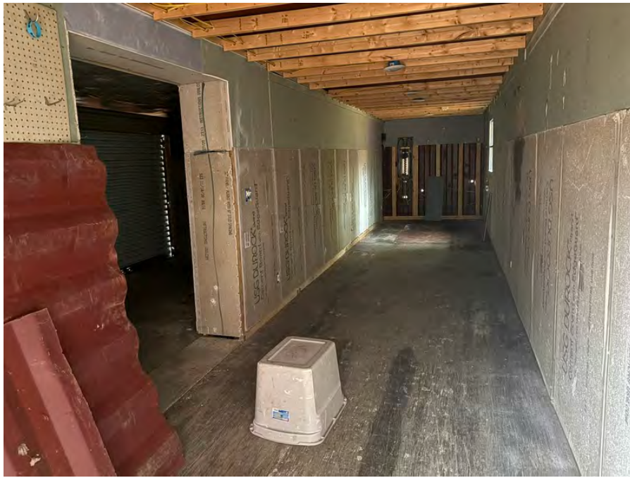
Photo 13 : View inside structure
